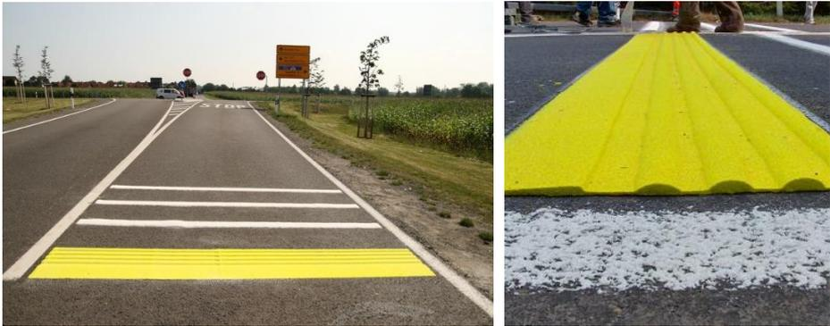
**Figure 3: Finished profile stripes<sup>1</sup>**
